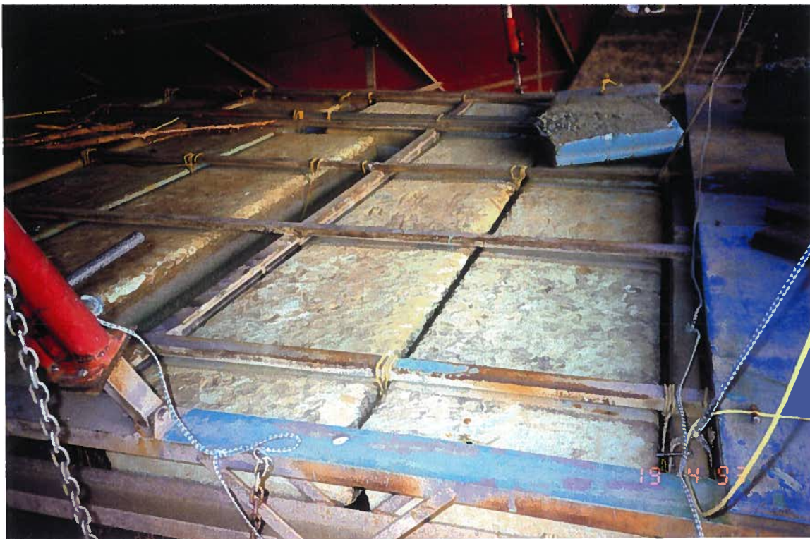
FLOTATION SHOWN TIED INTO PLACE.
