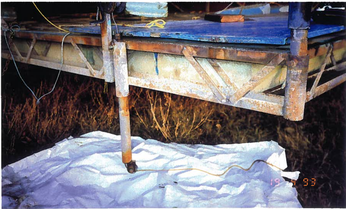
FRONT RIGHT WINCH WITH CABLE SLEEVE IN POSITION.
